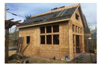
**SITE-BUILT/TRADITIONAL** The ADU is custom-built on your property with typical construction methods.
